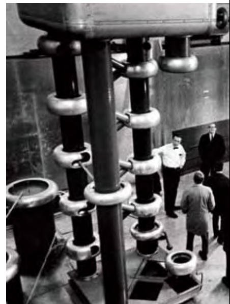
In 1969, Fermilab technicians set up a Cockcroft-Walton borrowed from Argonne National Laboratory to test Fermilab's pre-accelerating column and the first tank of the linear accelerator.
